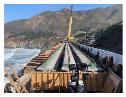
After a mid-December 2024 installation of concrete girders, crews will pour the concrete bridge deck for the southbound lane of the Rocky Creek viaduct during an overnight closure of Highway 1. Travelers will encounter a full closure of Highway 1 at Rocky Creek on Tuesday, Jan. 21, 2025, from 10 p.m.-6 a.m. (Caltrans)
